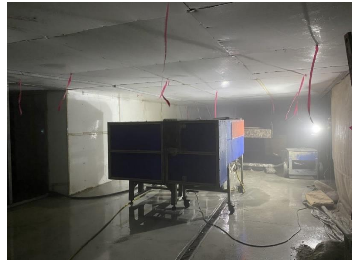
Dust Gallery after 15 Minute of Scrubber Operation
