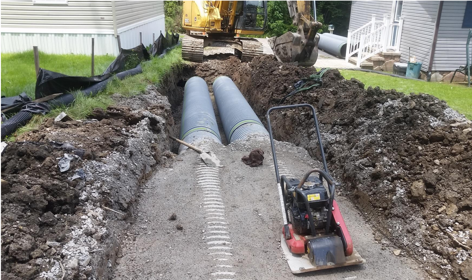
An example of an AML installed Drainage Culvert with Dense Grade Aggregate backfill.
