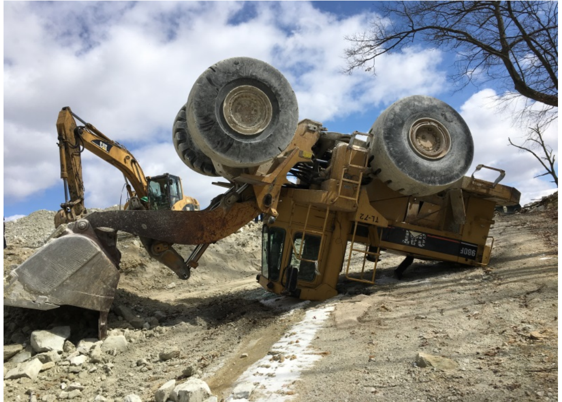
Loader operator saved by wearing seat belt
