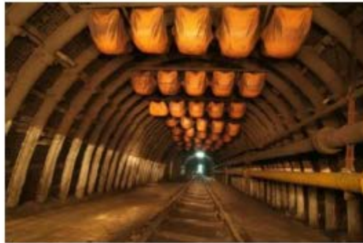
a) Passive barrier (Distributed/water)
