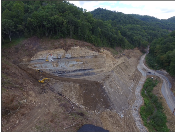
New No. 2 Gas Mine Face Up
