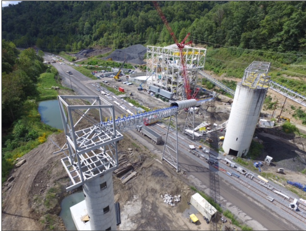
Raw Coal Silos, Preparation Plant & Clean Coal Stacking Tube
