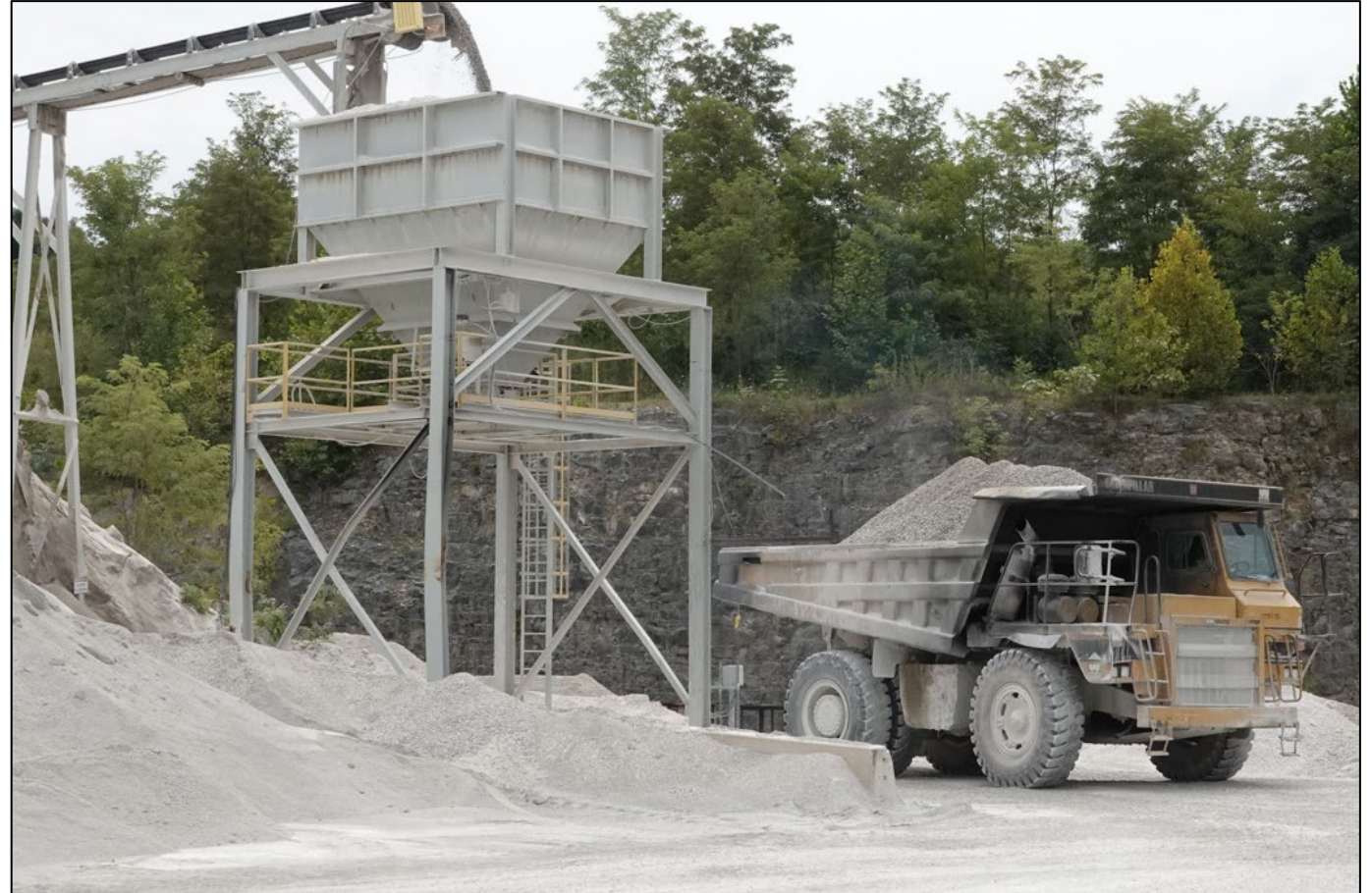
Photo: Truck loading with limestone gravel at central Kentucky quarry.
