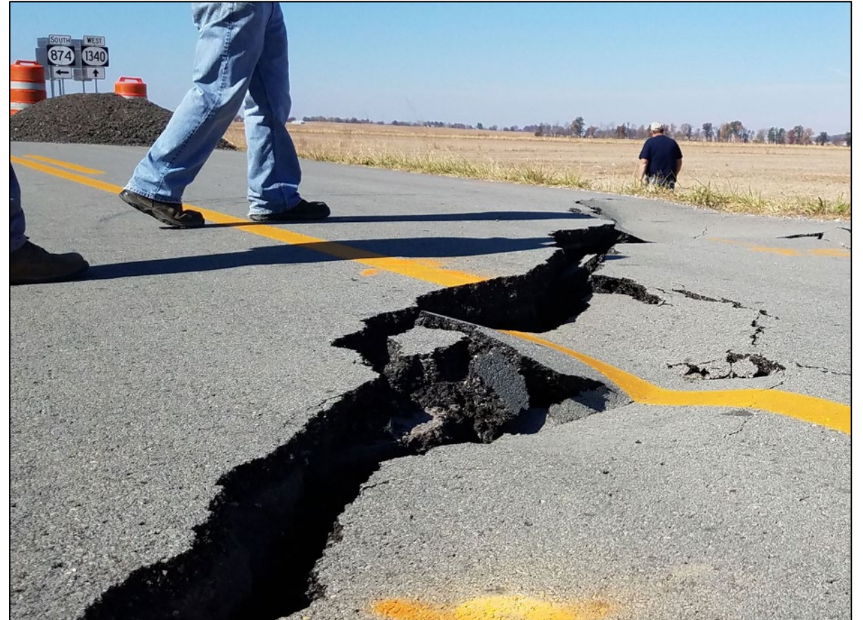
Photo: Subsidence across state road in western Kentucky.
