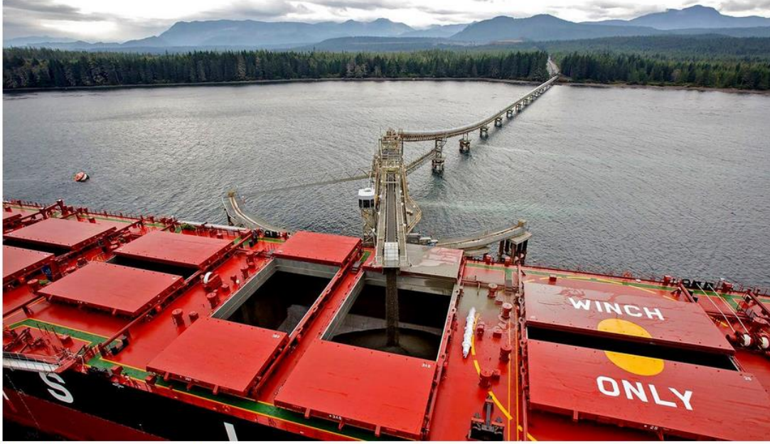
Conveyor belts stretching more than a mile from the Orca quarry on Vancouver Island in Canada carry gravel and sand to a ship off the coast of Port McNeill. (Polaris Materials)
